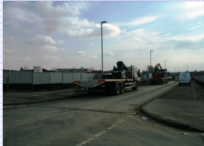
Thorpe Road New Build Housing Development site
