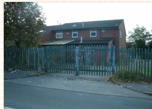
Site 24 – Broom Court
