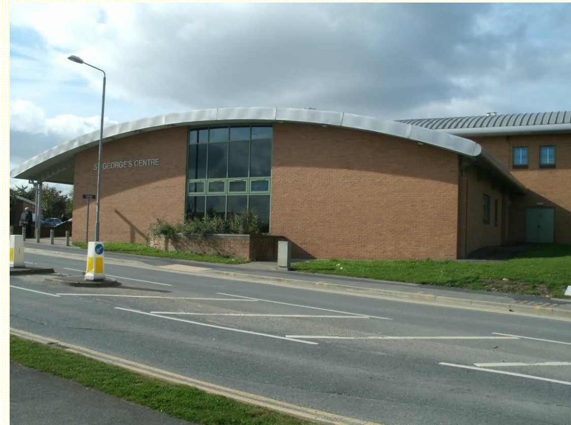
Well used community asset - St Georges Centre in Middleton
